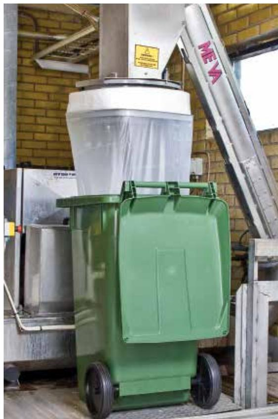
Staffanstorp Municipal Sewage Treatment Plant in Sweden has installed a Longopac Fill for the handling of screenings.
